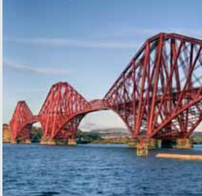
Forth Rail Bridge
